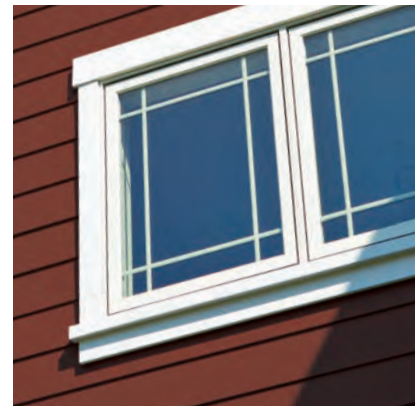
Window surrounds complete the curb-appealing picture.
