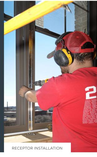
Receptor systems have long been used on job sites with aluminum windows, but now there is a customized solution for vinyl window projects. Harvey's aluminum receptor system simplifies and accelerates installation in projects with challenging existing conditions. This thermally broken product is used in place of interior/exterior stops, resulting in a cleaner look than traditional installations.
